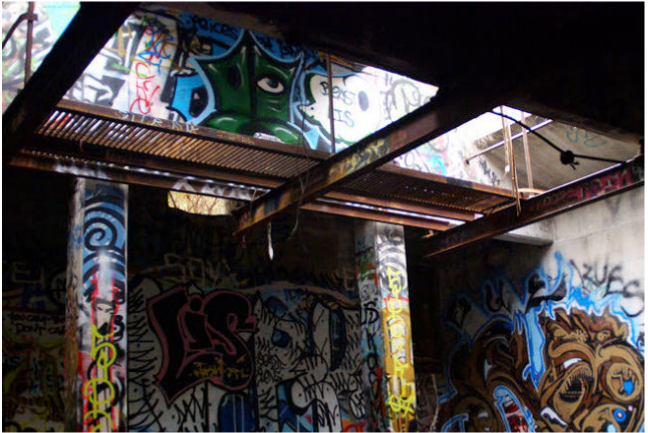
Murphy Ranch's generator station as it looks today.
